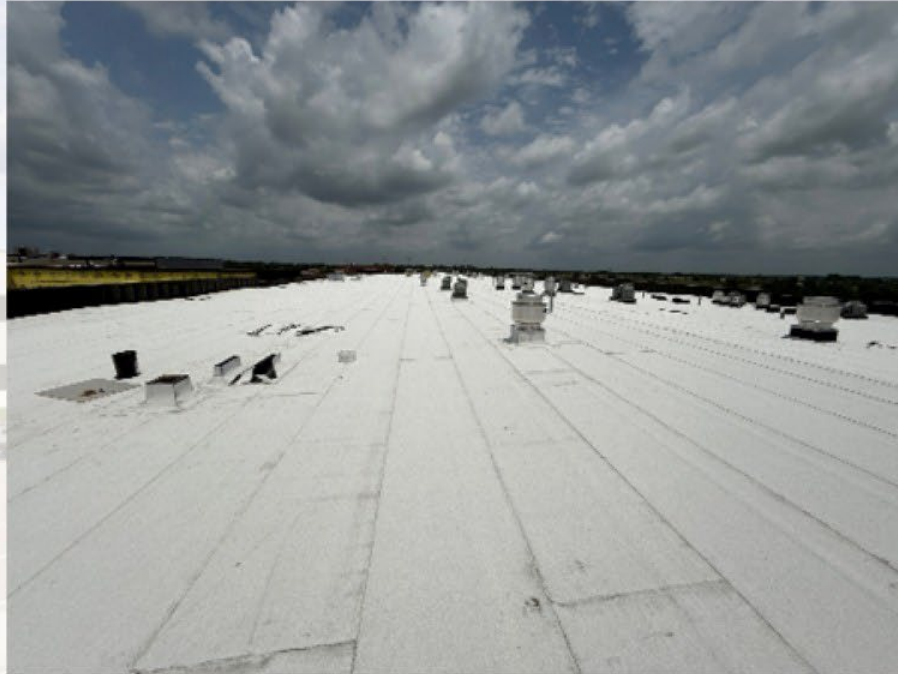
CLASSROOM WING ROOF
