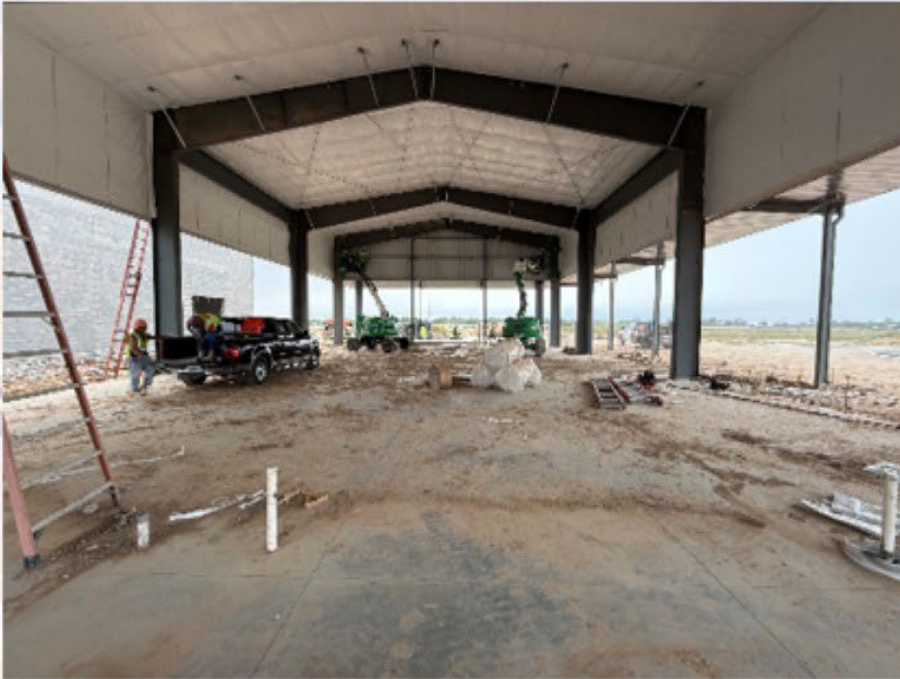
AG SHOP WITH EXTERIOR STORAGE
